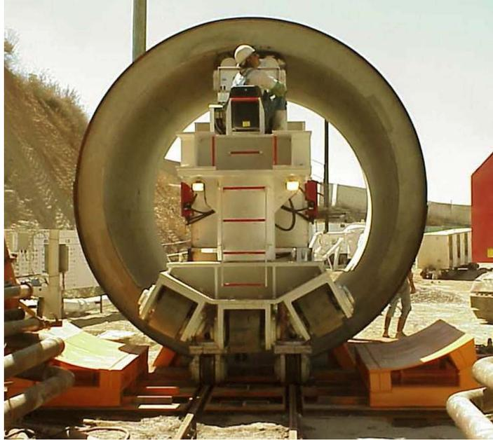
Figure 1. 144-in. Diameter Composite Wall Tunnel Liner
